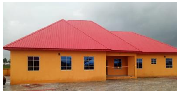
Front view of the newly commissioned Ilaje RDC Secretariat at Ode-Ugbo, Ondo State
